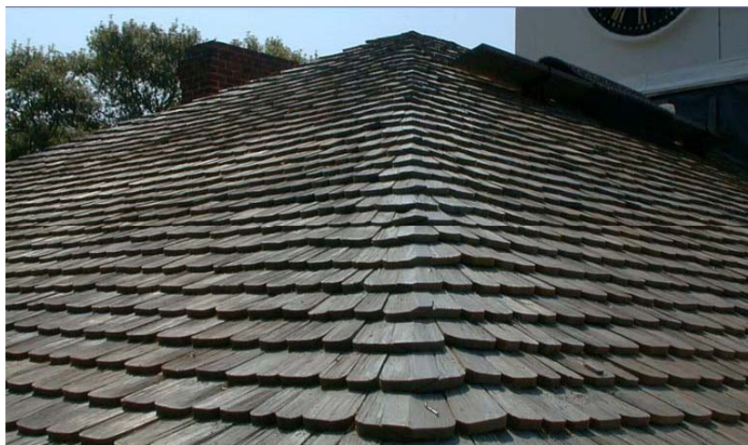
Figure 2 (Photo by Progressive Contractors, Inc.)
