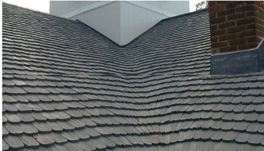
Figure 1 (Photo by Progressive Contractors, Inc.)
